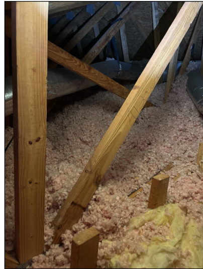
Insulation appears adequate.
