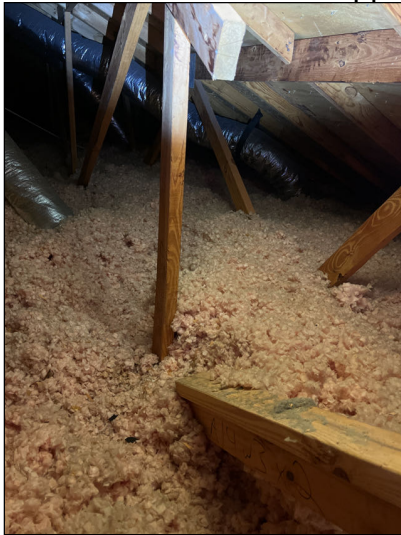
Insulation appears adequate.
